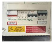
2. Turn off the main switch **Inverter Supply** in the meter box.
